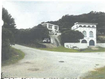
Street view of the houses directly across Milkwood Crescent from erf 13 on the left, high perched double storey house on erf 7 at the back right and triple storey house on erf 8 in the front facing Beach Crescent.
