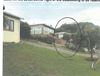
Street view of erf 13 right, with the neighbour's house erf 14 to the left, showing steep driveways with low density vegetation. The garage extension will have minimal impact when viewed from this angle.
