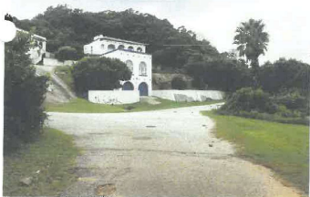
Street view looking up Beach Crescent to a neighbour's house and erf 13 left side. The photo shows the clear vehicular sight and view lines, the wide road reserves for parking and negotiating traffic
