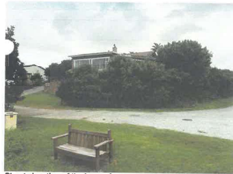
Street elevation of the house from across the street showing Milkwood Cresc starting on the right. The dense vegetation completely hides the Outbuilding and proposed garage extension
