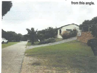
Street view looking westwards down Beach Crescent showing unimpeded sight lines and wide road reserves with erf 13 right
