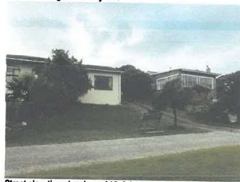
Street elevation showing erf 13 right and the neighbour's house, erf 14 on the left. Also showing wide road reserves and unimpeded views and sight lines for vehicles & pedestrians
